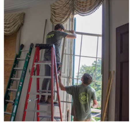
Lemon Hill Mansion window restoration
